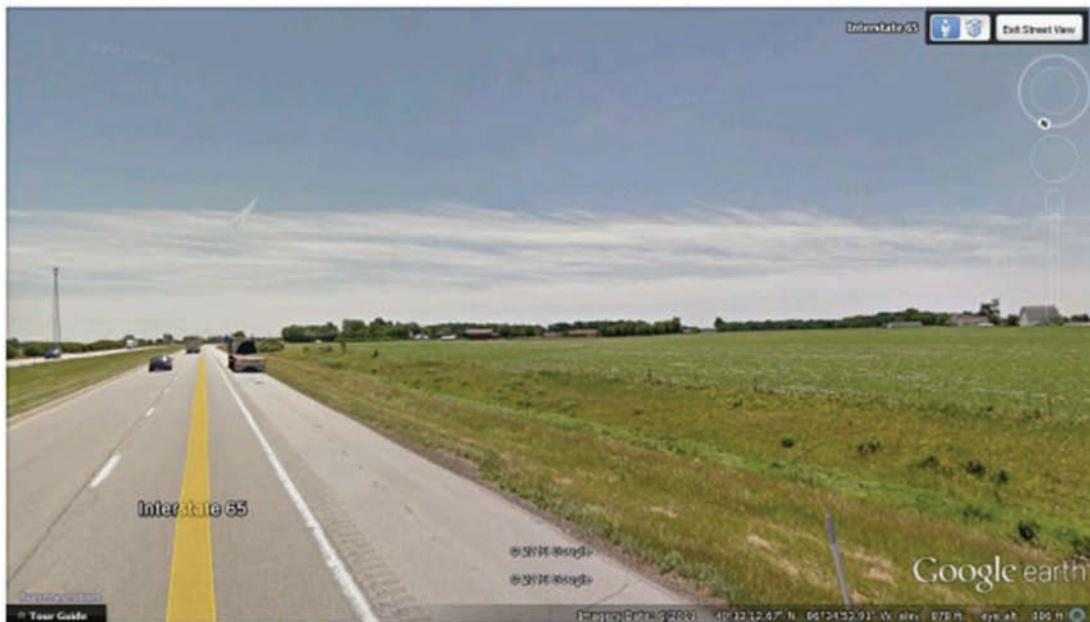
Clear zone greater than or equal to 30 ft; sideslope flatter than 1V:4H, recoverable.
