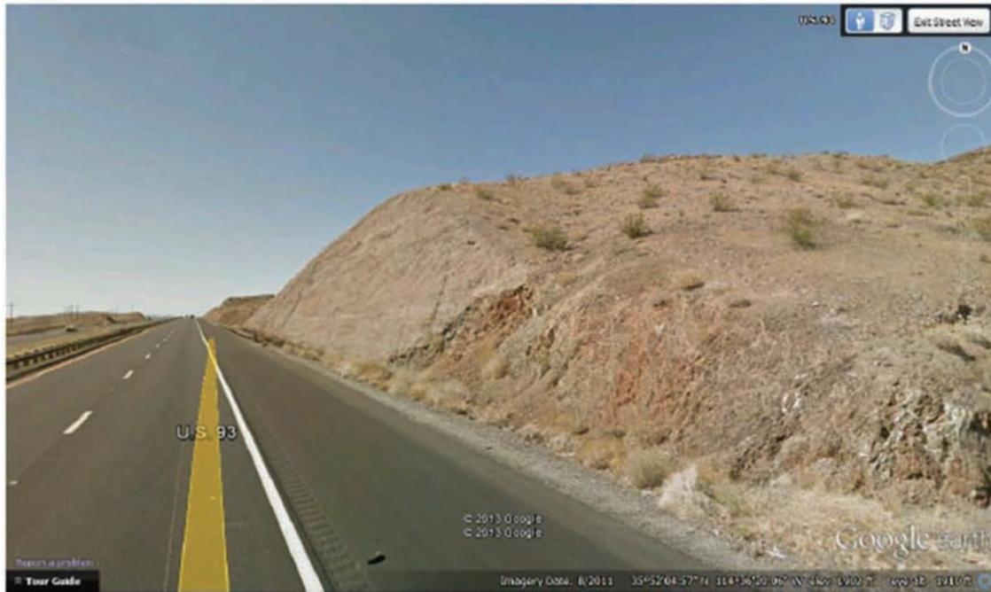
Clear zone less than or equal to 5 ft; sideslope about 1V:2H or steeper, non-recoverable with high likelihood of severe injuries from roadside crash.
