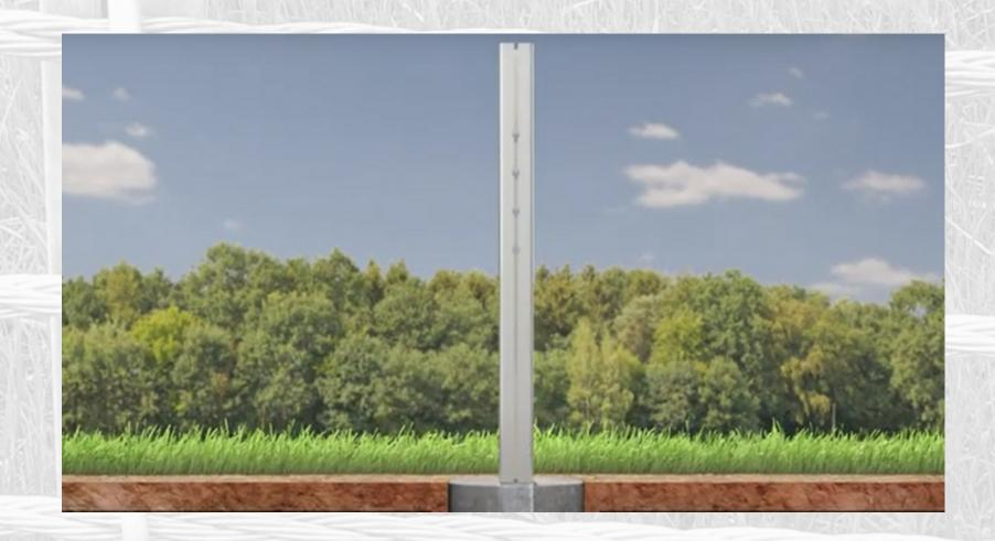
This socket should be installed on the opposite side of the cable of the TP1-4 socket. Be sure the 3-inch side of the socket is flush with the string line.
