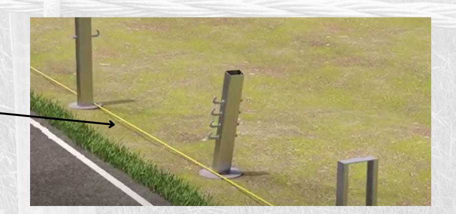
2) Locate the first line post socket at 14'6" from the last terminal post. Noting the socket needs to be on the opposite side of the string line of the TP4-4 post socket hole.
