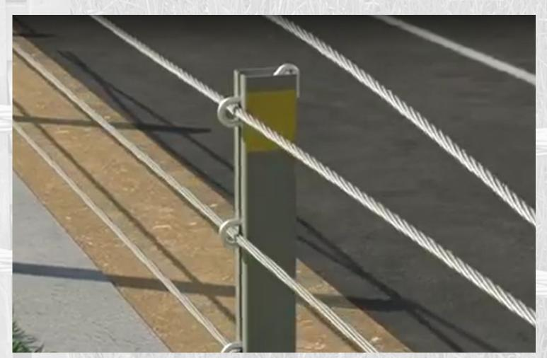
5) At the next post, the fourth cable will be placed on top of the hairpin. The top two cables will alternate going through the hairpin. They should never twist with the free cable at the post resting on top of the hairpin. After all the cables are installed, the fourth cable should be taken up to the appropriate tension.
