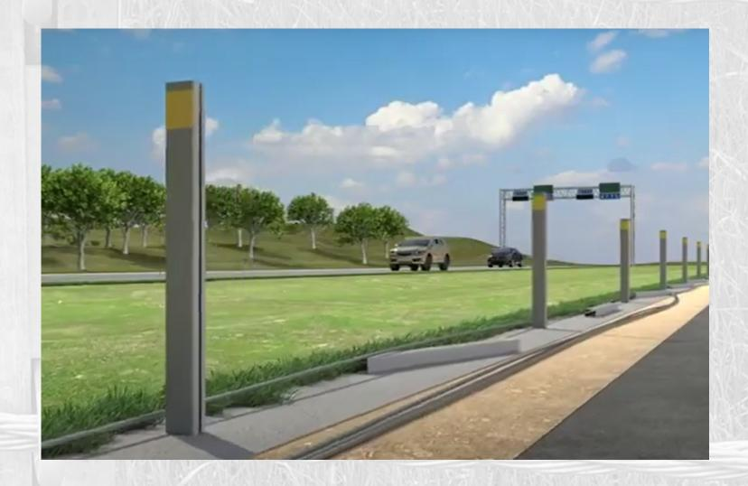
2) Hang three cables throughout the system utilizing a hairpin and lock plate. The fourth cable can remain on the ground.
