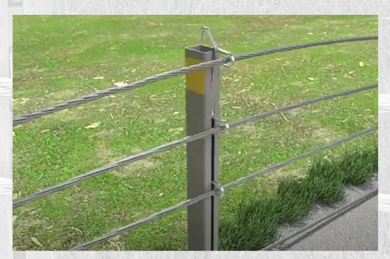
This process is best performed with a cable hanging device to keep the 3 cables in the correct order.
